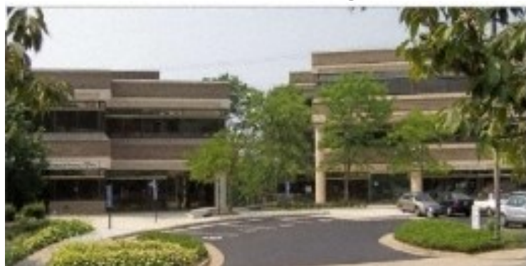
Front of Building
